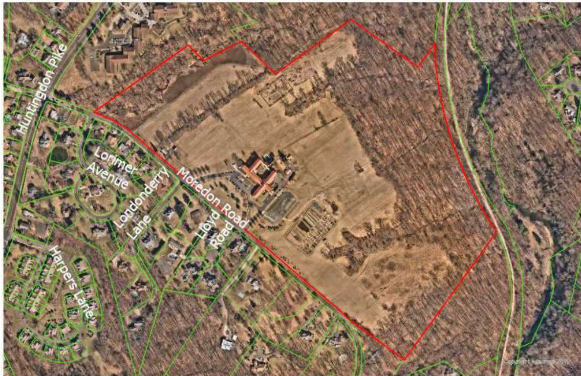
Solar Panel Array at 521 Moredon Road MCPC#220113001
