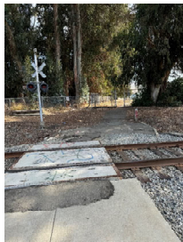
Existing: Lack of safety features at Tennyson High School Pedestrian Crossing (Hayward)
