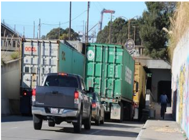
Truck stuck at the 7th Street underpass.
