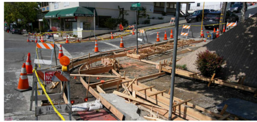
City of Piedmont – Grand Avenue Bike/Ped and ADA Improvements
