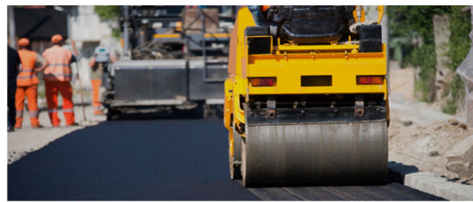
City of Hayward – Street Rehabilitation
