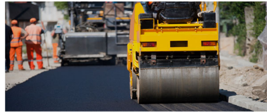
City of Hayward – Street Rehabilitation
