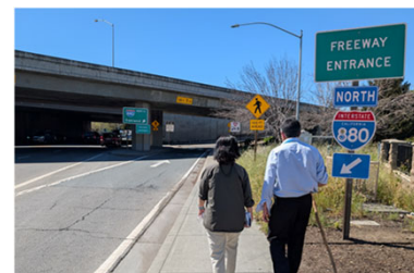
Lewelling Blvd & I-880 NB on-ramp
