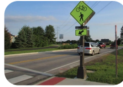
Flashing Beacons (RRFBs)
