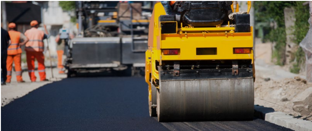
City of Hayward – Street Rehabilitation
