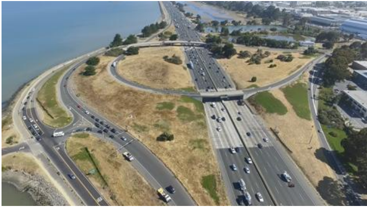
Aerial view of I-80/Ashby Avenue (SR-13) interchange.
