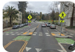
Flashing beacons/ Ped signals
