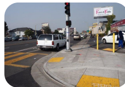
ADA ramp and signal upgrades
