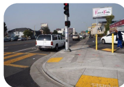
ADA ramp upgrades
