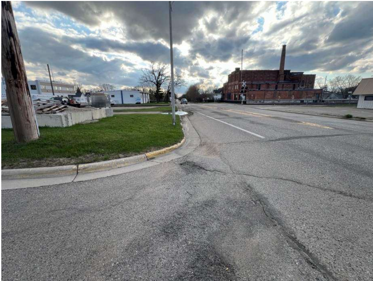
Figure 2: Gutter Line on South Side of Street, Looking West
