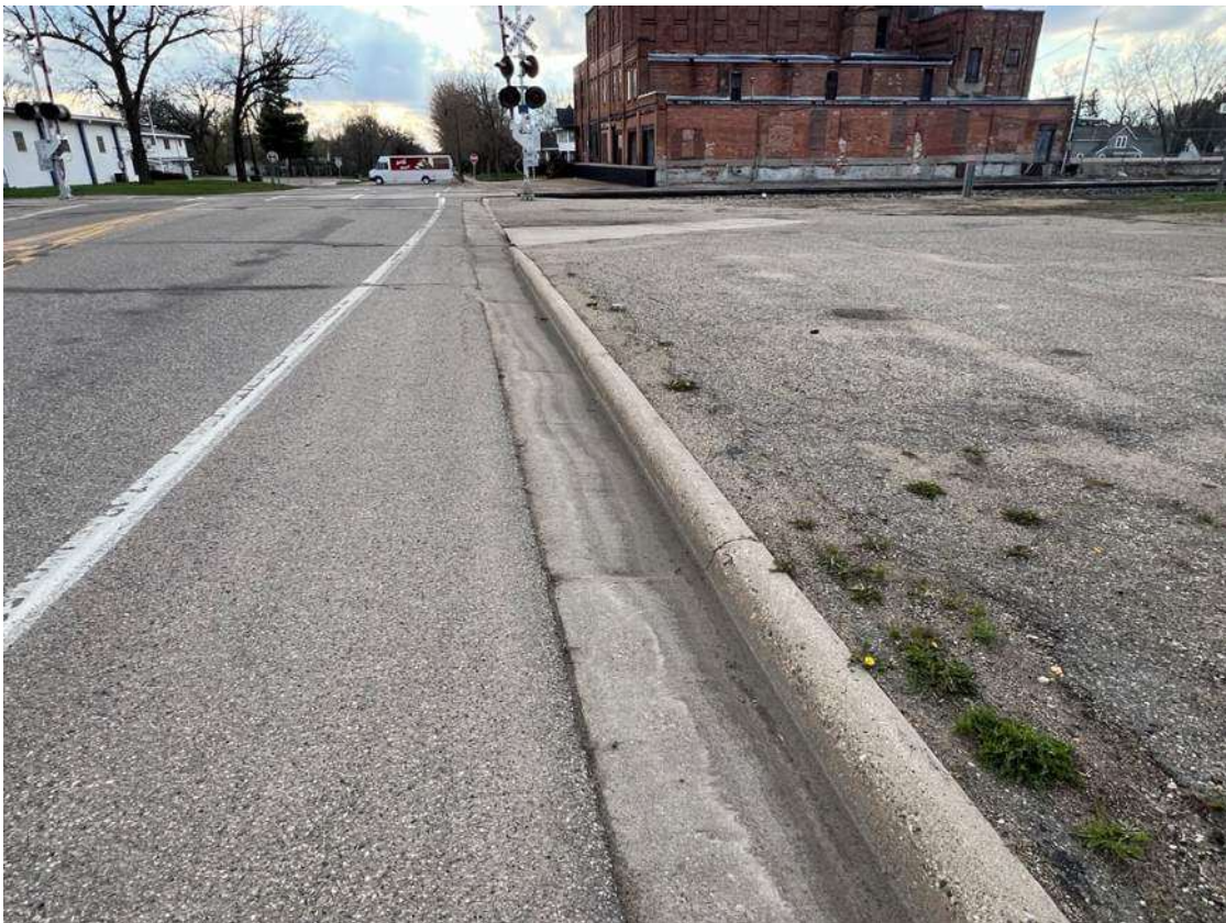
Figure 1: North Side of Street, Looking West
