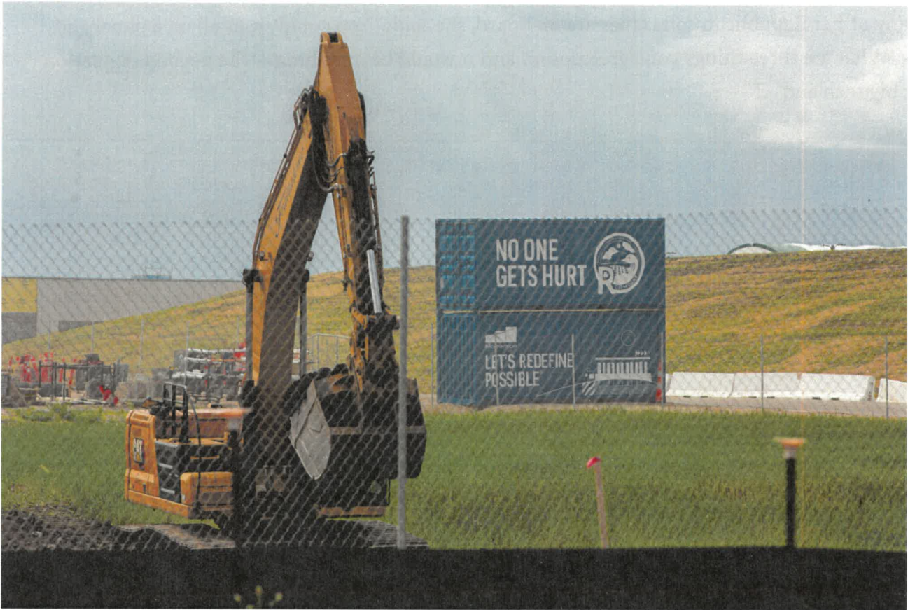
📷 Construction continues on the sprawling Rosemount Data Center on land bought by Meta near Dakota County Technical College, shown Thursday, May 29, 2025. (Photo by Nicole Neri/Minnesota Reformer)
