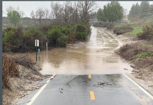
Aliso Creek flooding during a storm in 2019. Courtesy of City of Aliso Viejo – Local Government Facebook Page
