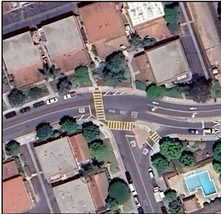
Forced Turn Barrier. Source: Google Earth 2025, City of San Juan Capistrano.
