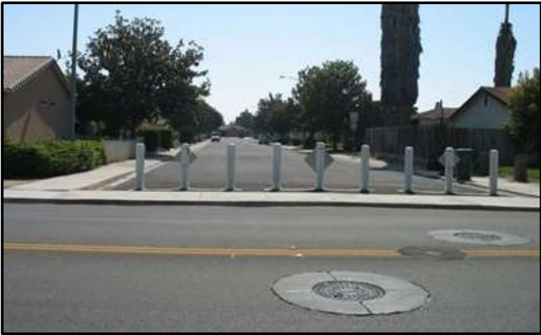
Full Closure. Source: Caltrans.
