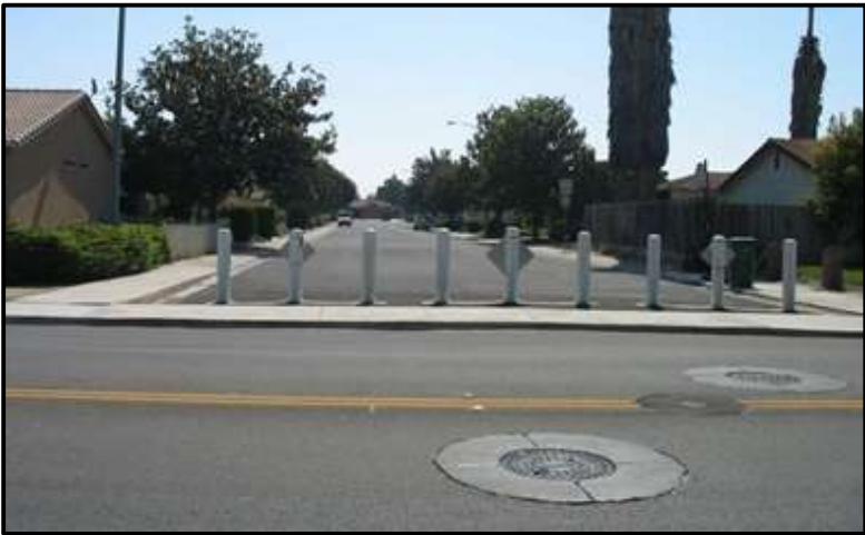
Full Closure. Source: Caltrans.
