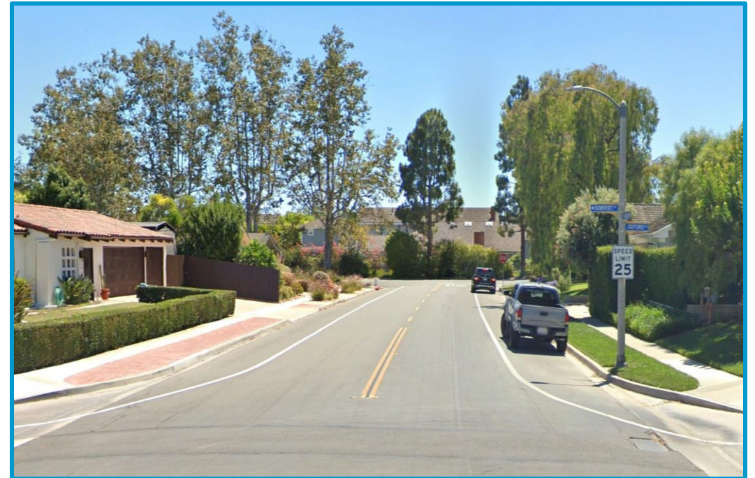
Signing & Striping. City of Newport Beach.
