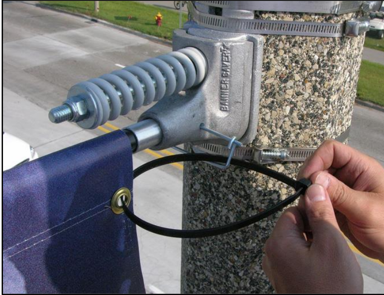
Figure 1 – Method of Securing Banner to Pole Bracket
