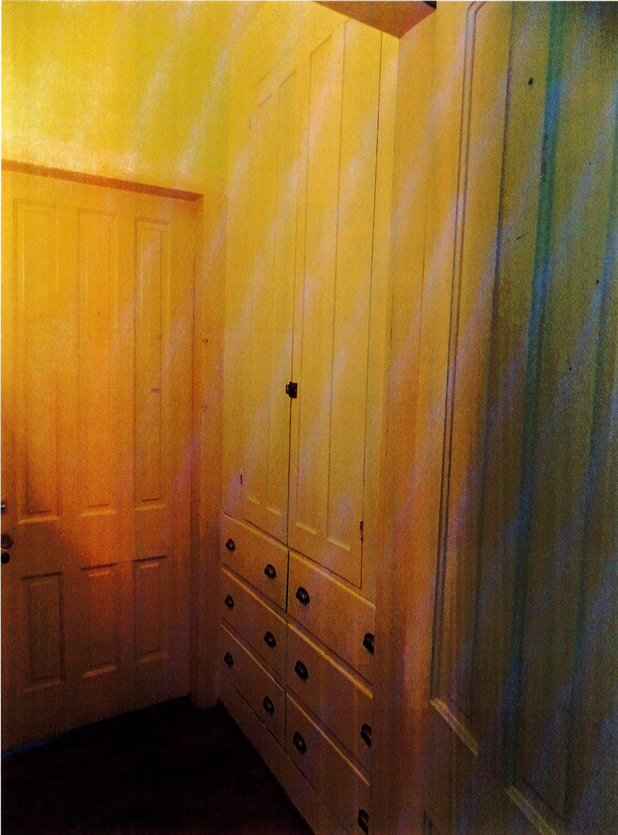
Built-in cabinets, second floor hallway
