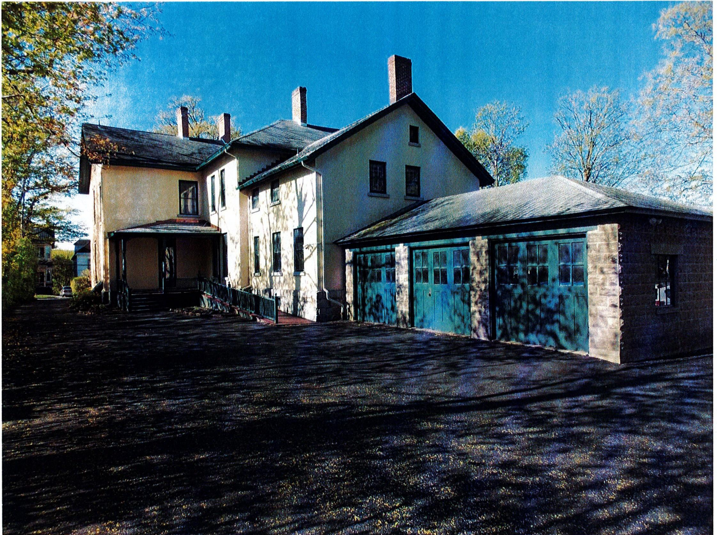
View of additions and attached garage
