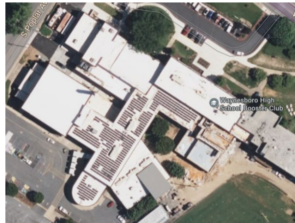
Figure 1: Photovoltaic Panels on Waynesboro High School in Waynesboro, VA
