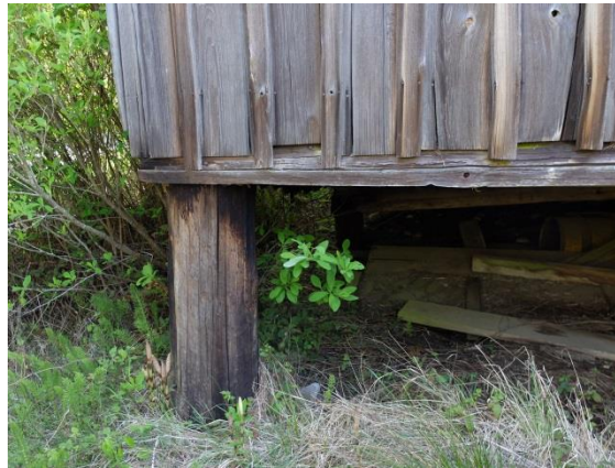
Figure 4e. Imbedded pole columns.
