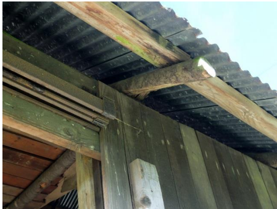
Figure 4d. Pole rafters and corrugated roof.
