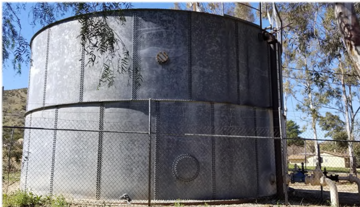
Figure 8.9: High Valleys Tank
