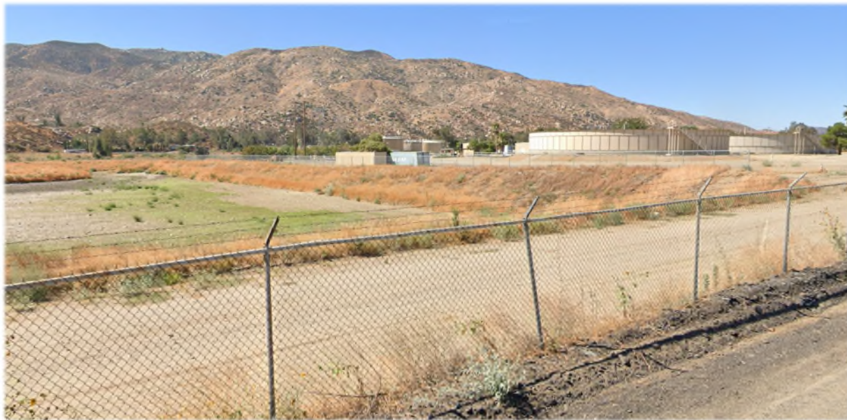
Figure 3.10: Spreading Grounds at WWTP
