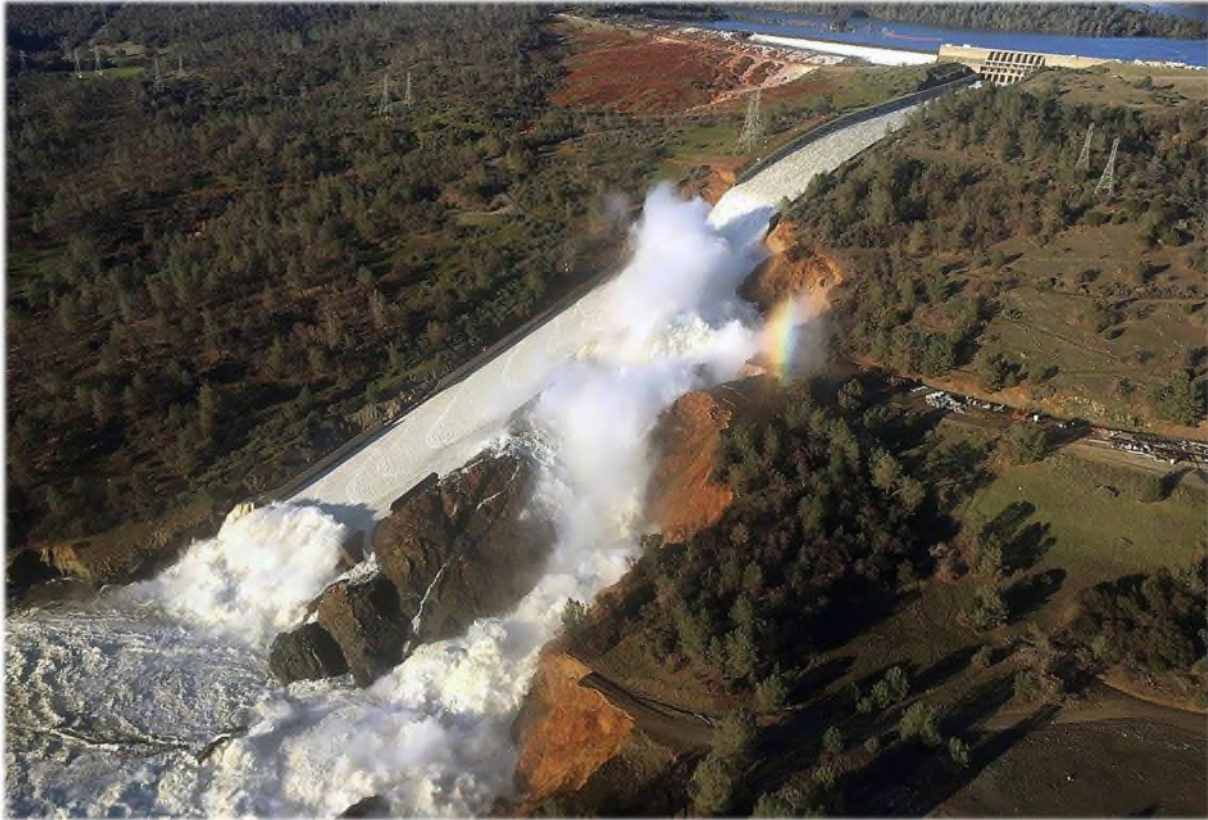
Figure 8.1: Lake Oroville Failure (February 2017)
