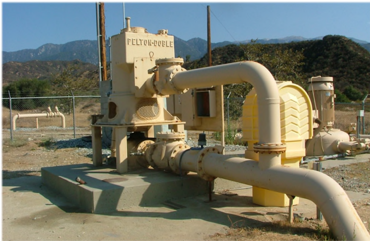
Figure 8.7: Pelton Wheel Pump
