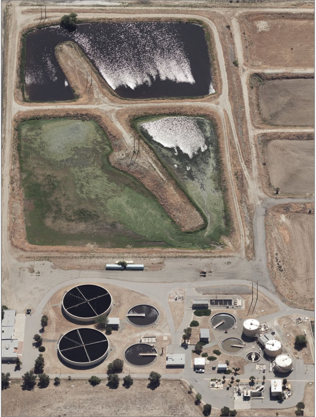
Figure 4.3: City of Banning WWTP and Percolation Ponds
