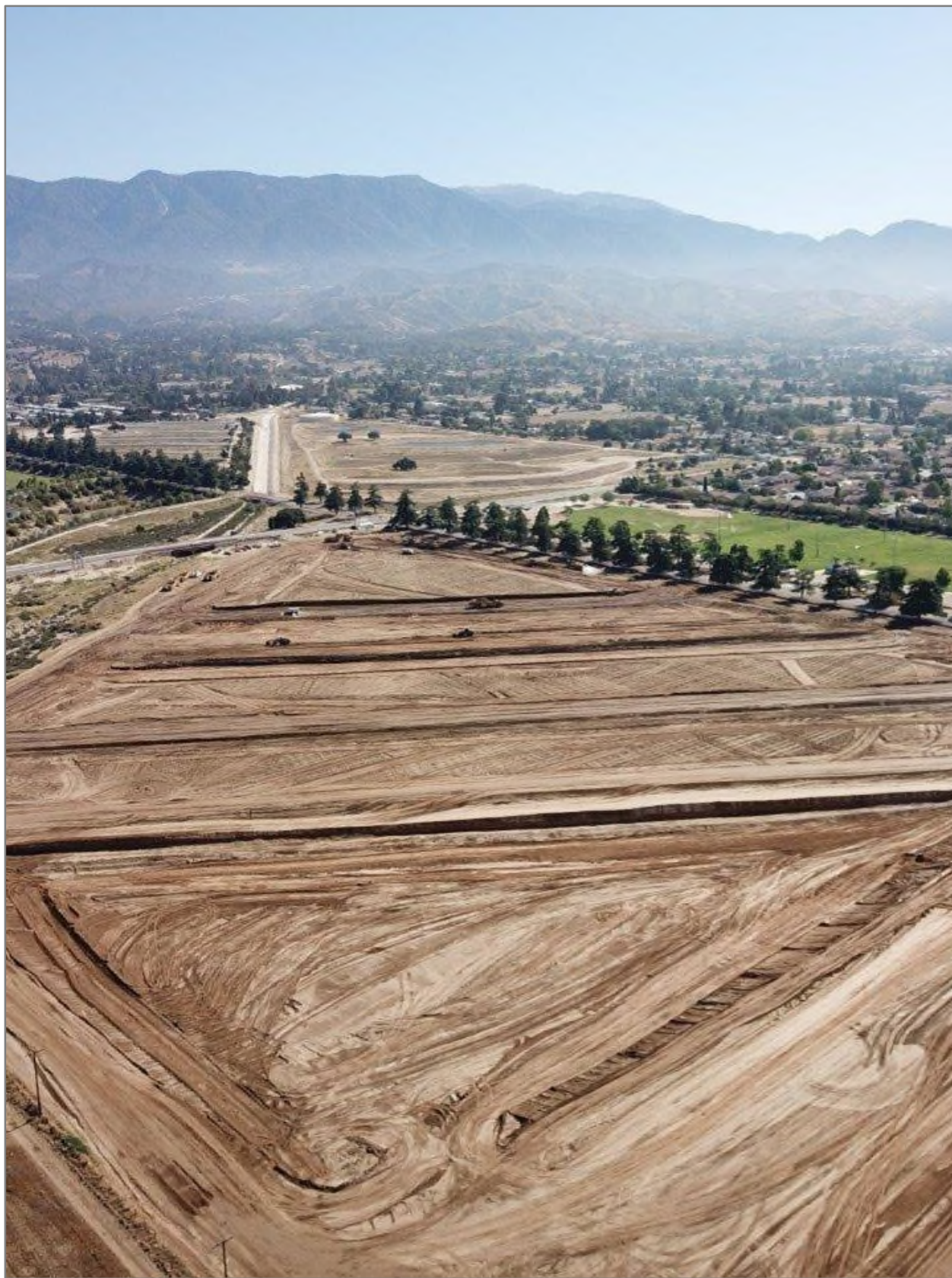
Figure 3.6: Brookside Recharge Facility
