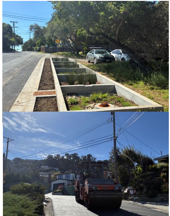
Figure 1 (top) - New bioretention area constructed on Alameda de las Pulgas Figure 2 (bottom) – Finish rolling on King
