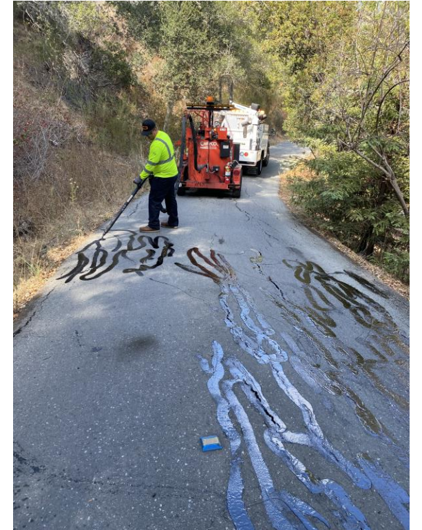
Crack Sealing
