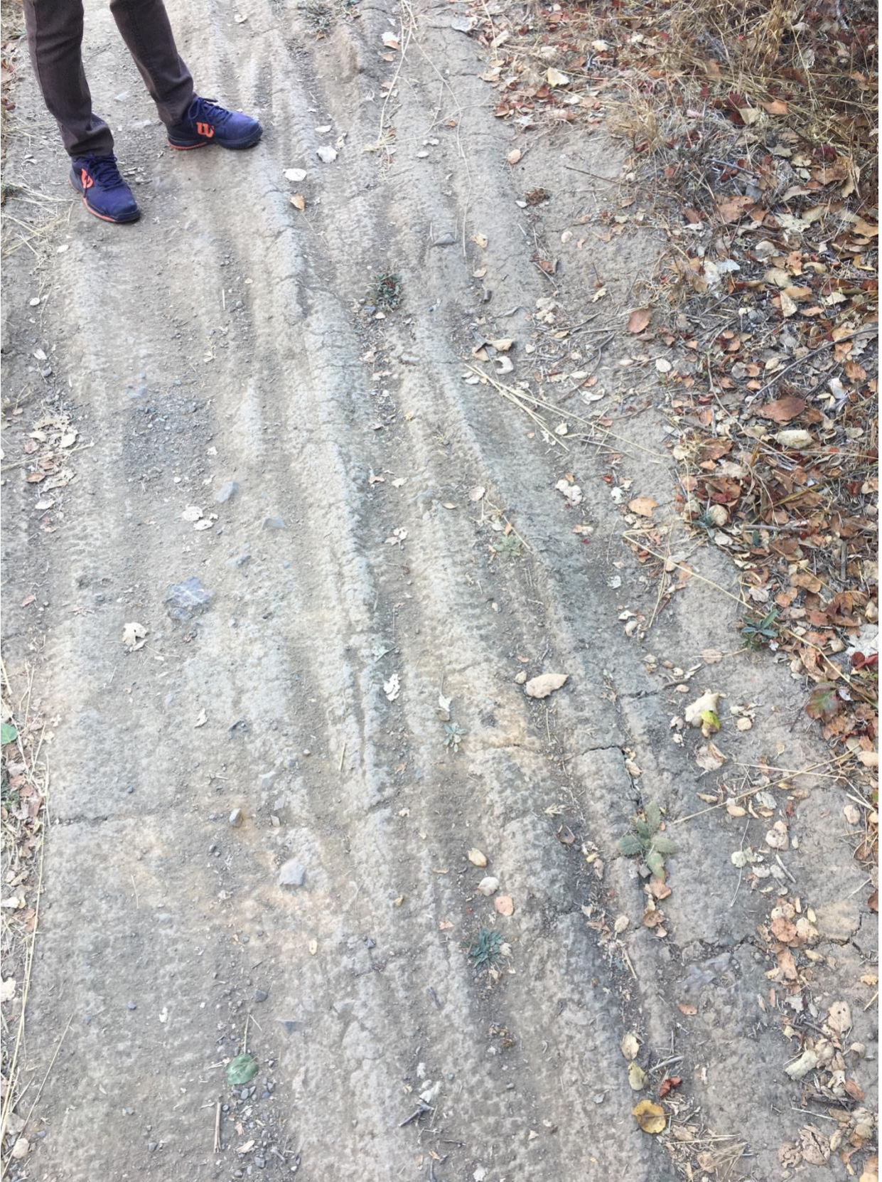
Figure 8. Tire ruts on the Brooks hillside trail.
