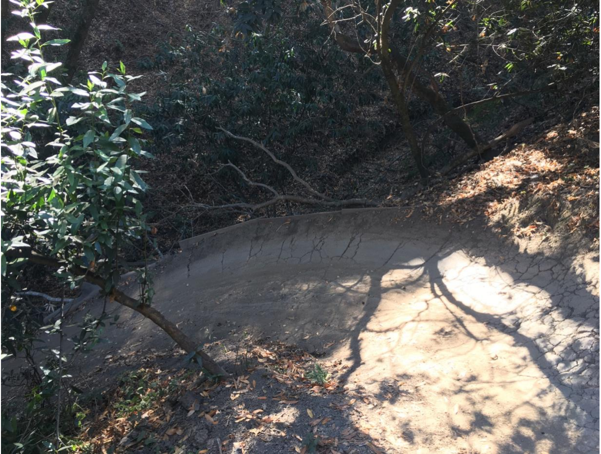
Figure 2. Technical trail feature (descending turn) installed on the Brooks hillside trail.
