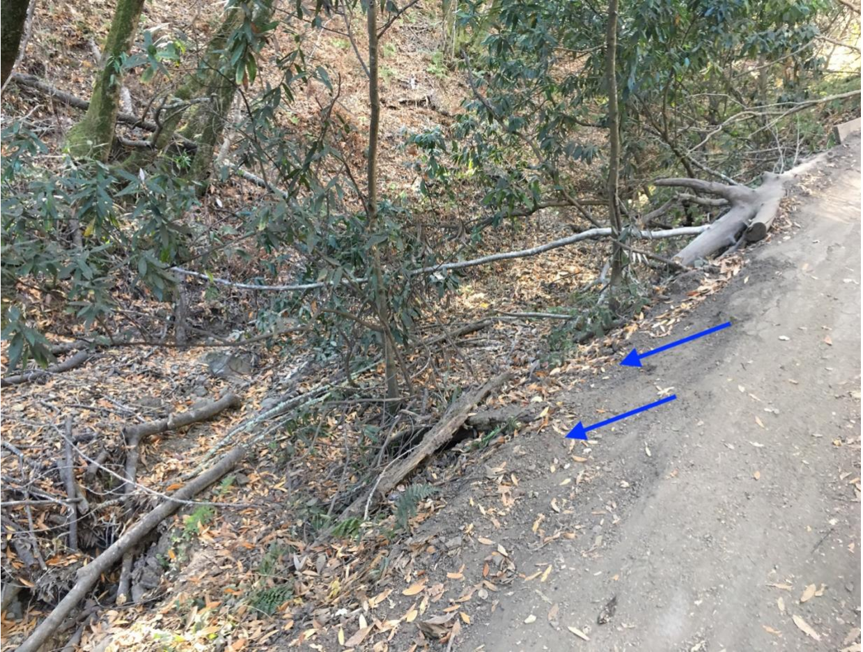
Figure 9. Trail damage along the Canyon Creek Trail. Blue arrows depict direction of sediment transfer into the adjacent ephemeral stream.
