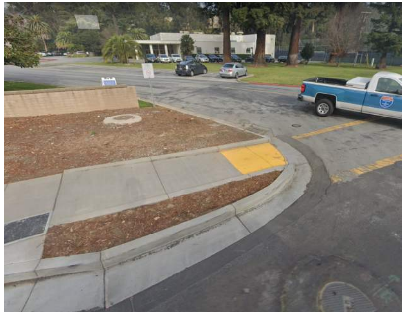
"After" fully ADA compliant curb ramp transition to new concrete sidewalk
