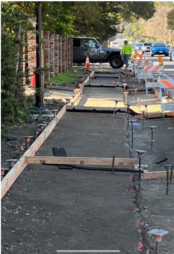
During sidewalk construction at 1500 block of Ralston Avenue
