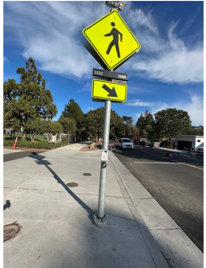
"After" driveway entrance and RRFB at Barrett Community Center
