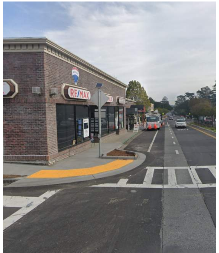
"After" revised curb ramp with bulb-out to reduce pedestrian crossing distance
