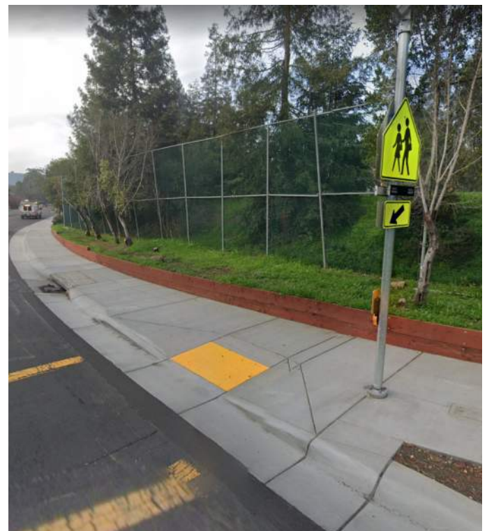
"After" fully ADA compliant curb ramp transition to new concrete sidewalk with new RRFB at Chula Vista
