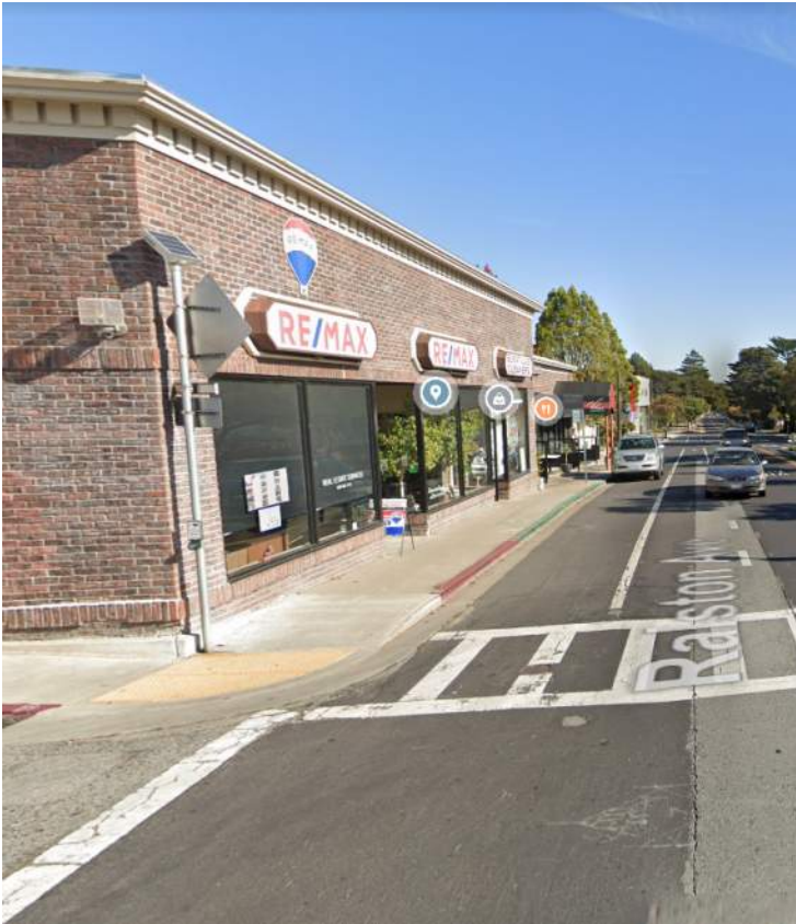
"Before" curb ramp at Villa and Ralston Ave intersection
