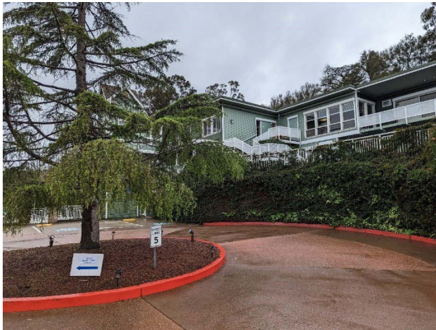
Existing facility looking south from 900 6 th Avenue parking lot (Erdman 2023).
