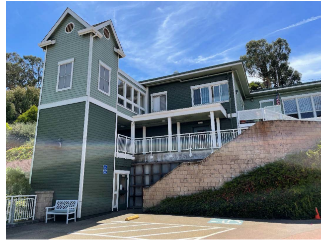
Existing facility with 1998 elevator addition (photo left), looking southwest from 900 6 th Avenue parking lot (Erdman 2022).
