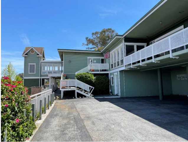
Existing skilled nursing facility looking southeast from Hill St (Erdman 2022).
