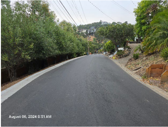
Figure 2 - Typical roadway conditions on project following completion.
