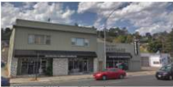
A1 Site A - SW from El Camino Existing adjacent structures
