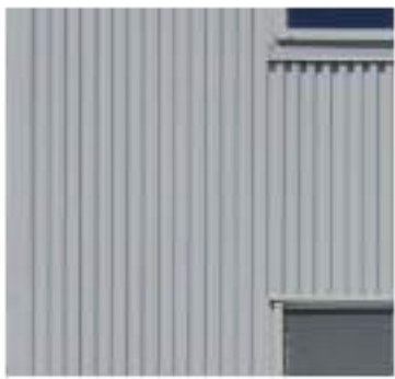
1. CORRUGATED METAL SIDING
