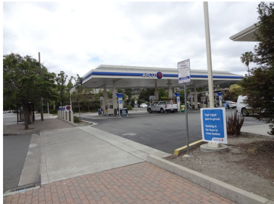
Most of the hazardous materials sites in Belmont are Leaking Underground Storage Tanks (LUSTs).
