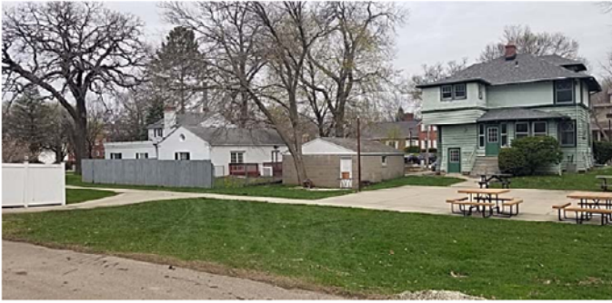
Houses at 749 and 706 Emerson to be Demolished
