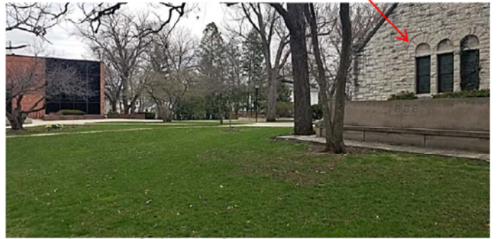
West Elevation of Library at future new entrance
