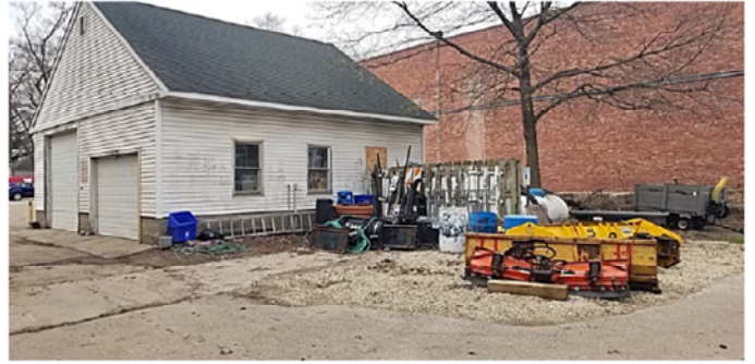
Garage at 732 Church to be Demolished
