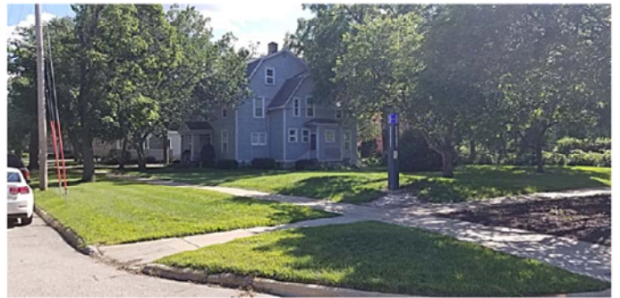
House at 742 Church Street to be demolished
