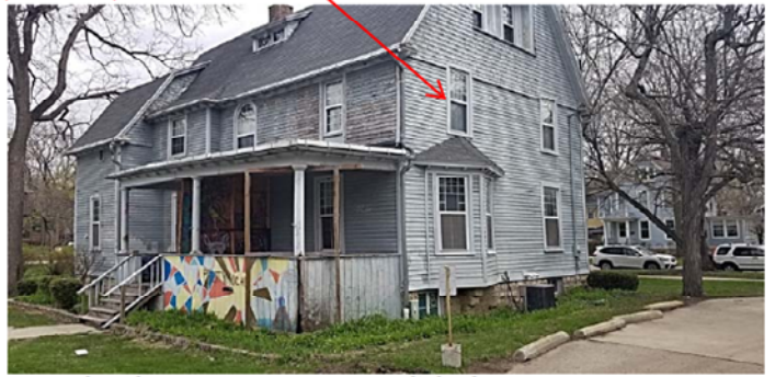
742 Church St. House To Be Demolished
