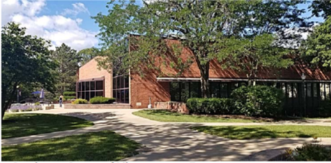
Southwest Corner of Library at new Entrance
