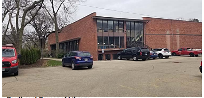
Southeast Corner of Library
