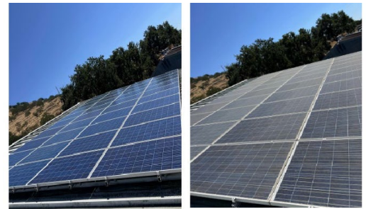
Example of a pre- and post- wash service results
