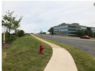
Bridge looking east over Normandale Boulevard.
