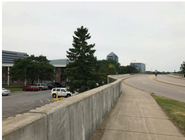
Bridge looking west over Normandale Boulevard.
