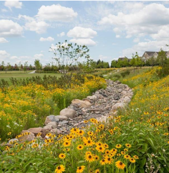
3 Stormwater Infiltration Basins
