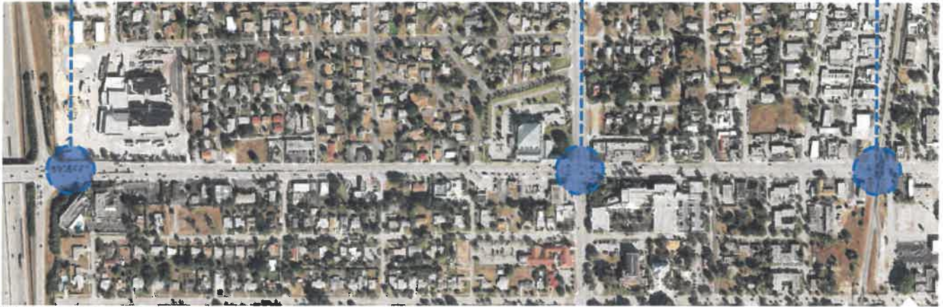
Figure 14: Intersection enhancements on Boynton Beach Blvd.
