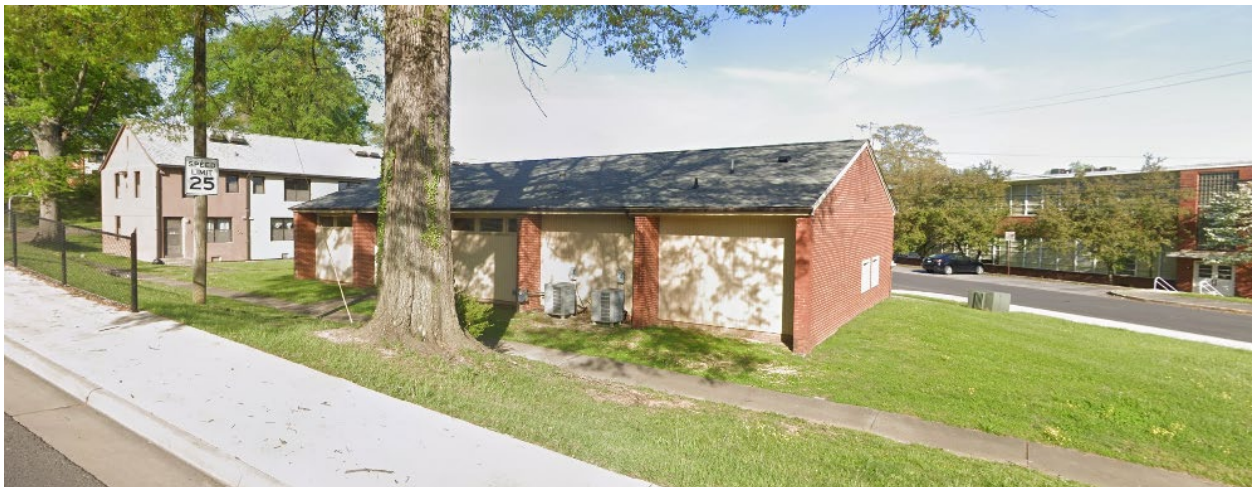
View of building from Lee Highway side
