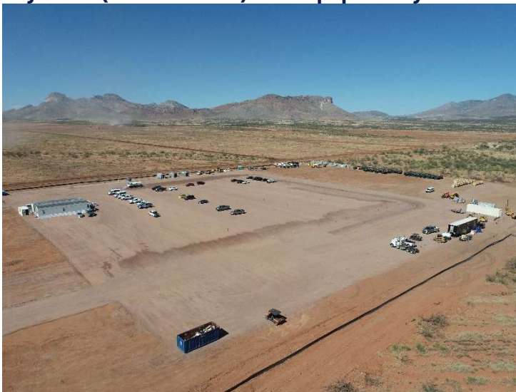
Typical laydown yard
