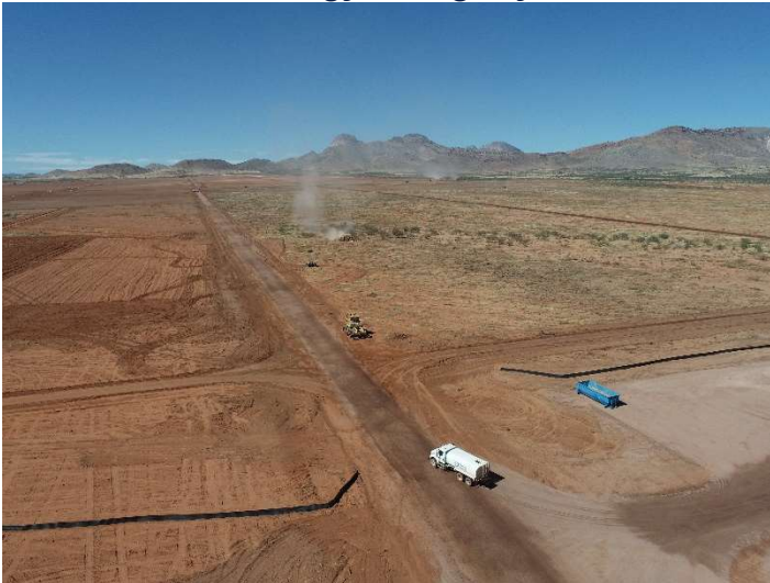
Typical access road constructed of compacted native material
