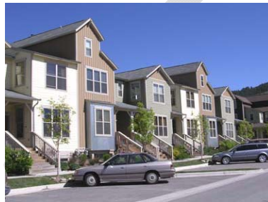
Figure 5.7-B: Examples of Building Articulation and Architectural Variety
