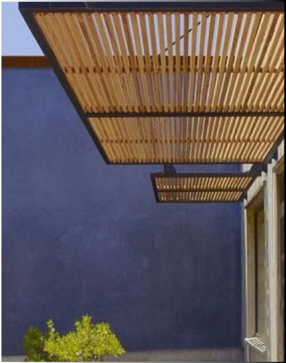
M-7 Tube Steel Trellises + Tiebacks
