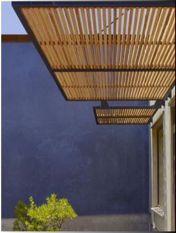
M-7 Tube Steel Trellises + Tiebacks
