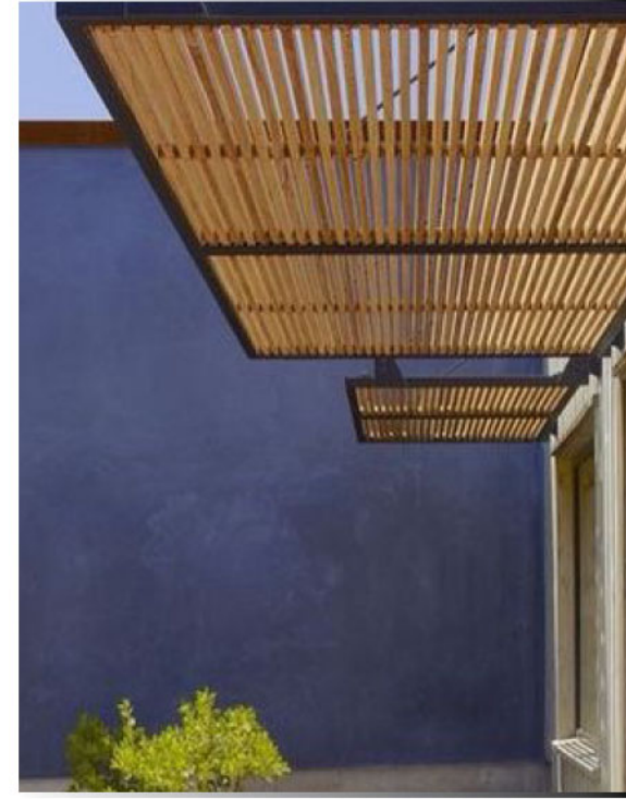
M-7 Tube Steel Trellises + Tiebacks
