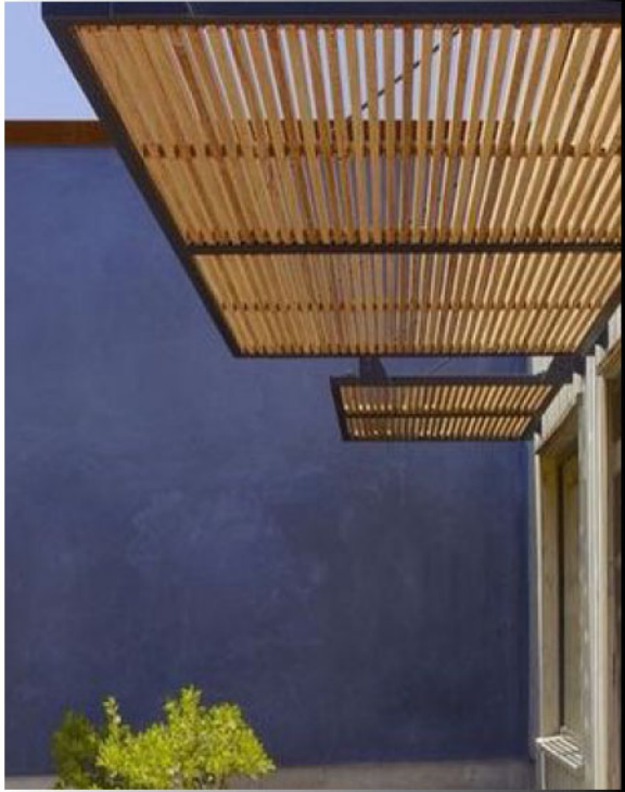
M-7 Tube Steel Trellises + Tiebacks
