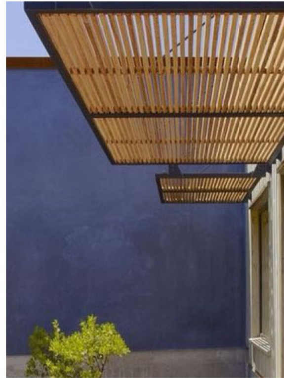
M-7 Tube Steel Trellises + Tiebacks
