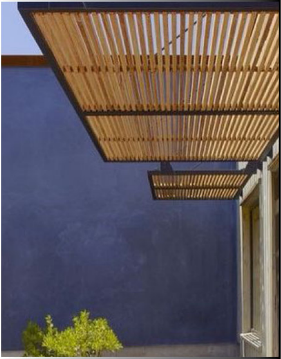
M-7 Tube Steel Trellises + Tiebacks
