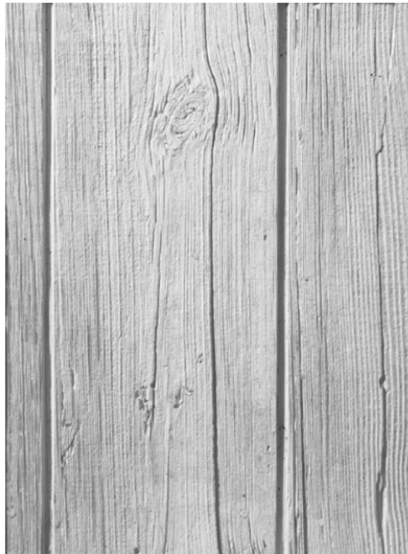
CONC-1 Tilt-up Concrete with Board Formed Formliner Texture
