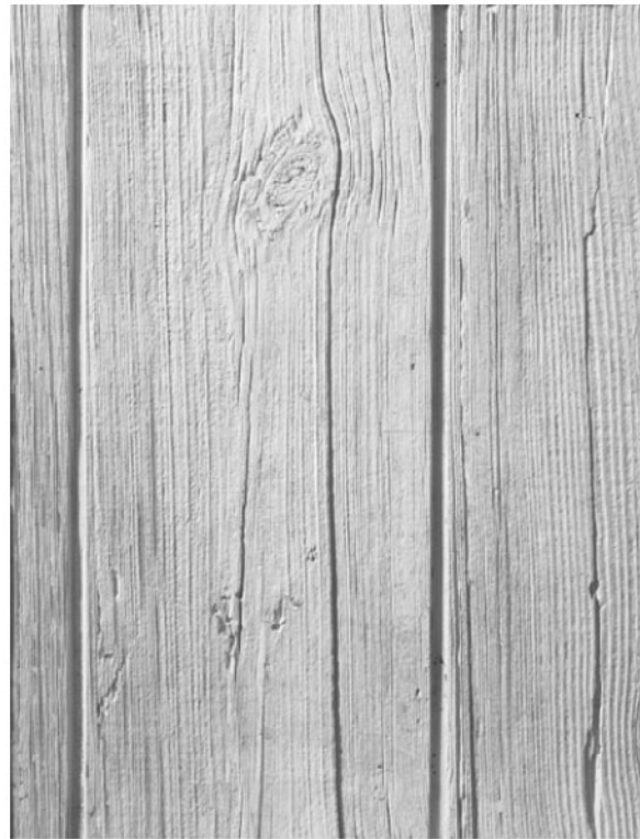
CONC-1 Tilt-up Concrete with Board Formed Formliner Texture
