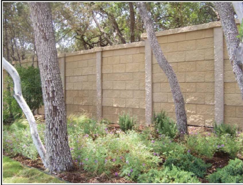
Split-Face CMU Style Concrete Fence
