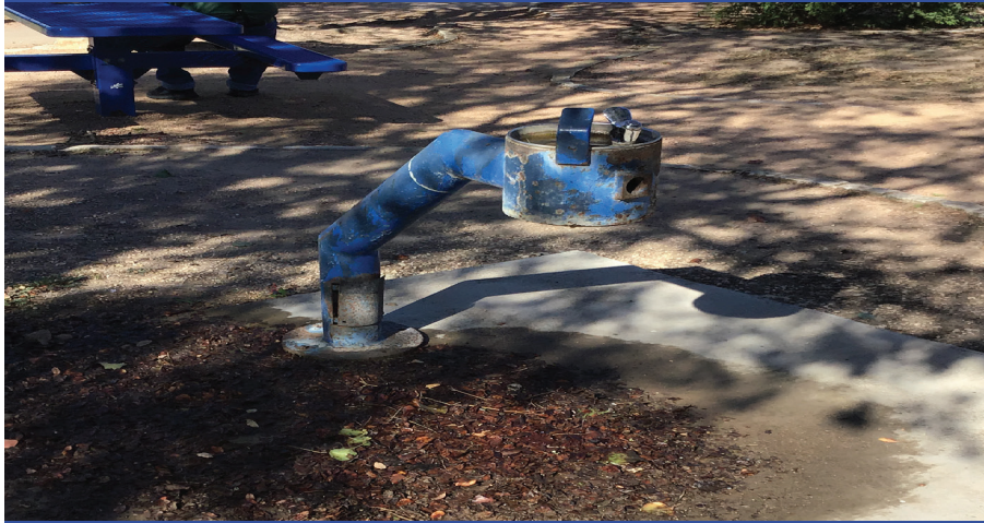
The water fountain in Bradfield Park is in need of replacement.
