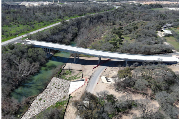
New bridge over Onion Creek connecting Jack C. Hays Trail to Cole Springs Road.
