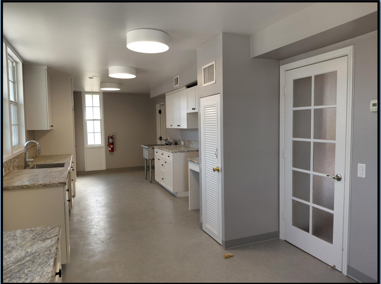
New Kitchen– Coquina Hall
