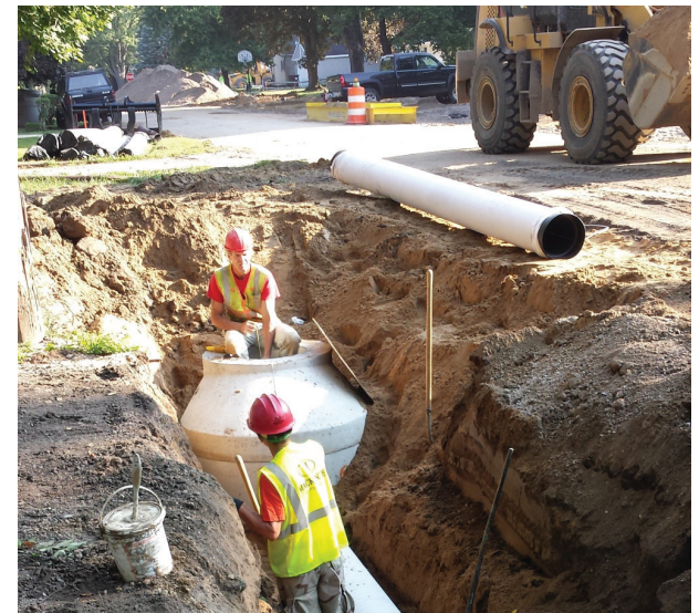
Pipeline being laid along a street
