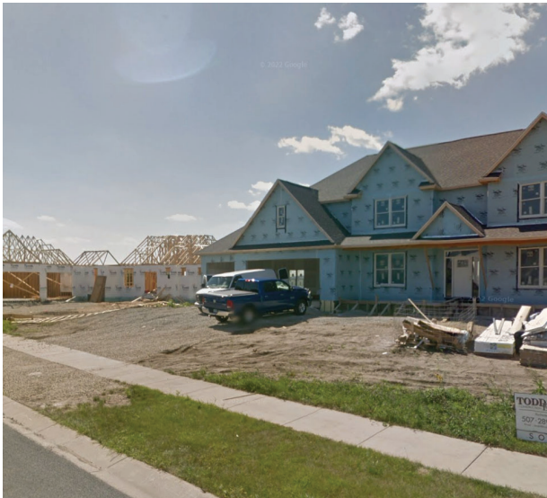
New homes under construction in Byron
