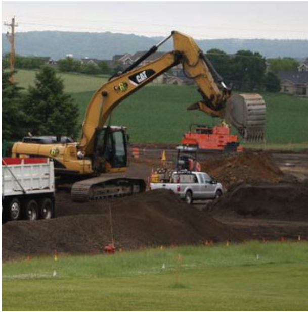
A roadway under construction
