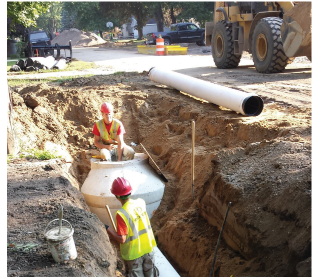
Pipeline being laid along a street
