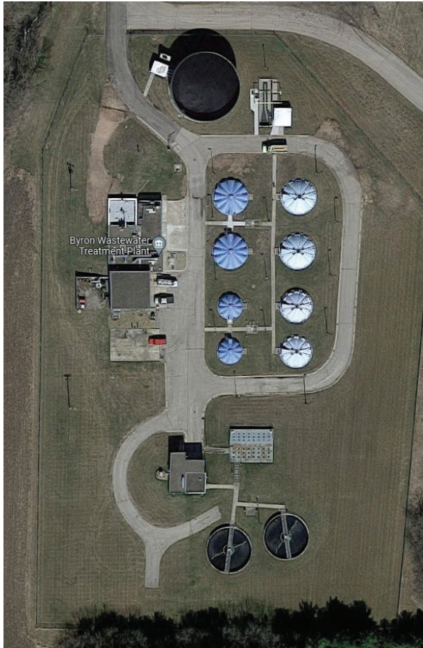
Byron Waste Water Treatment Plant
