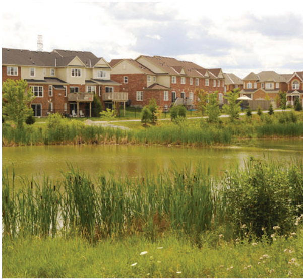
Stormwater pond by residential development
