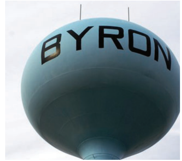
Byron water tower
