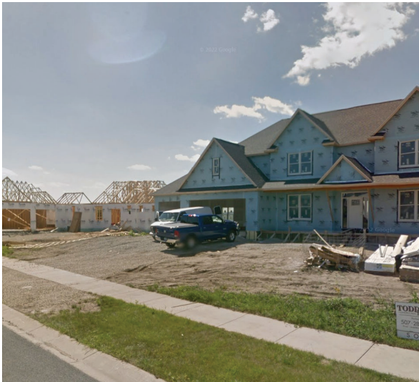
New homes under construction in Byron
