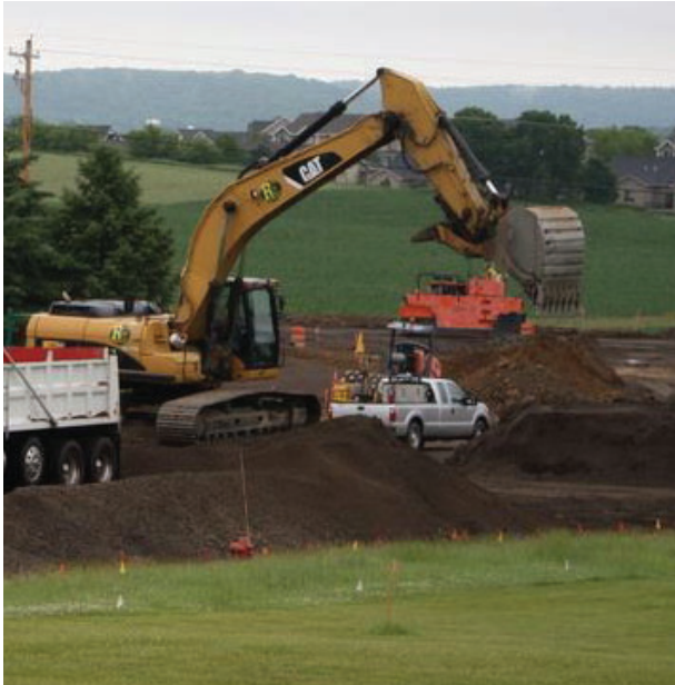
A roadway under construction
