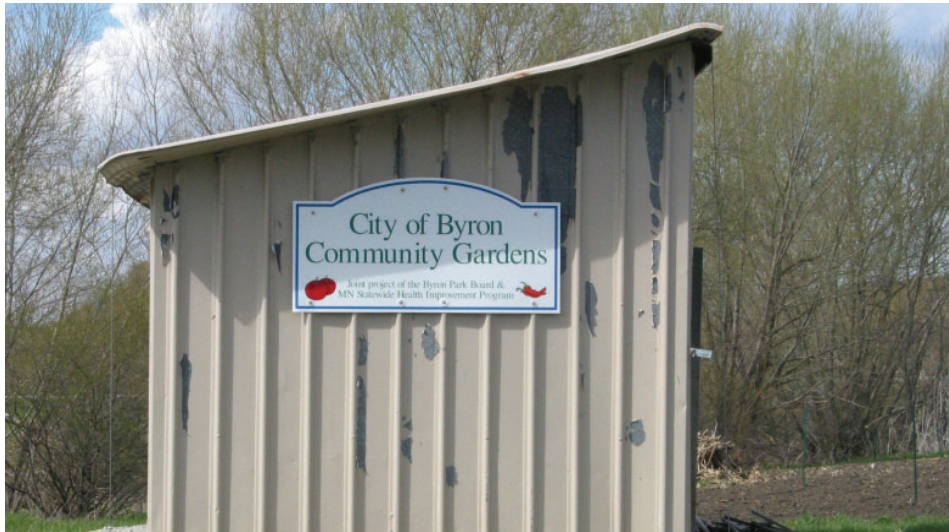
Community garden shed
