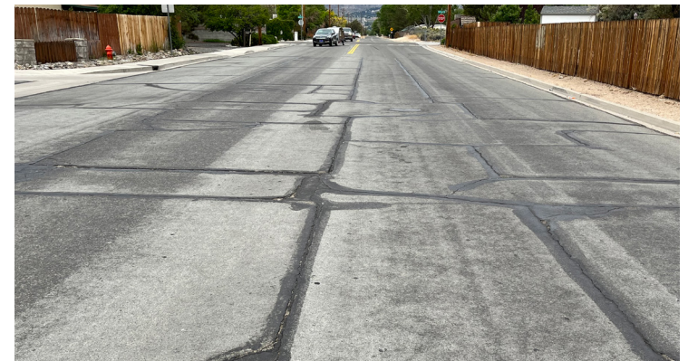
Figure 17: Example of a “Fair” pavement condition
