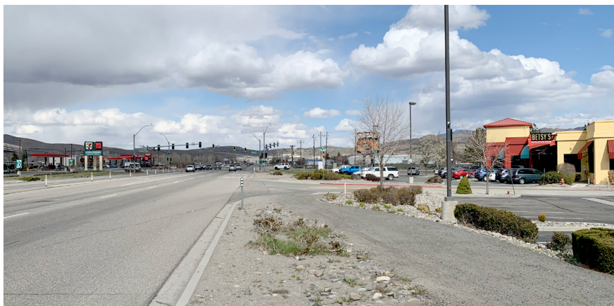
Multiuse path on US 50. Does not meet design standards; loose gravel on asphalt is a hazard.
