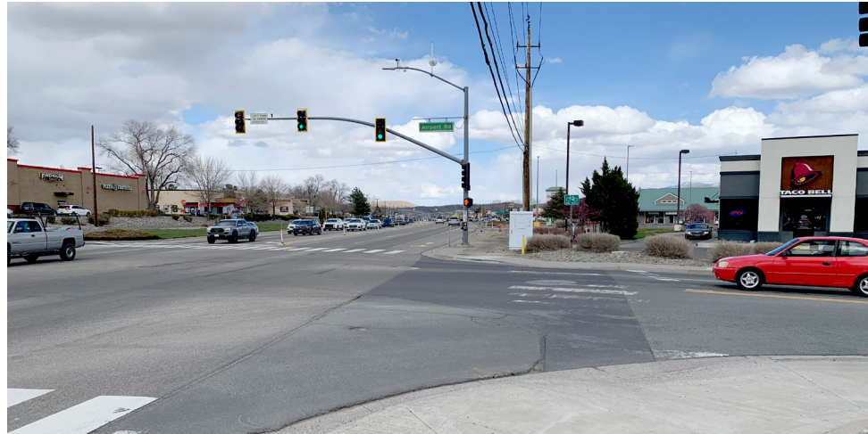
Intersection of US 50 and Airport Road. Inconsistent sidewalk, faded crosswalk, gap in connectivity.
