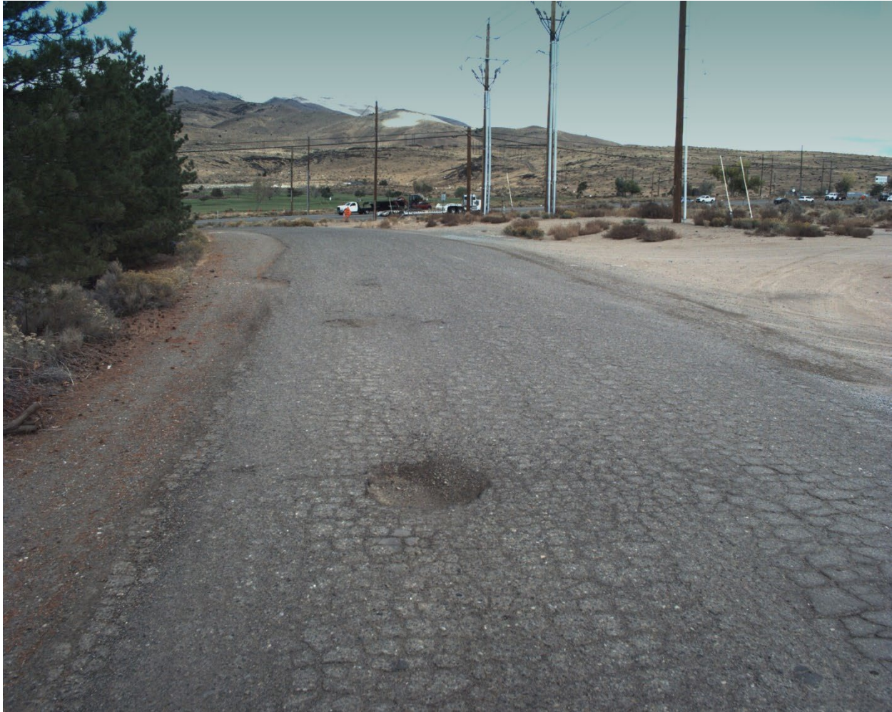
Figure 11. Pavement in Failed condition category (PCI 10–0).
