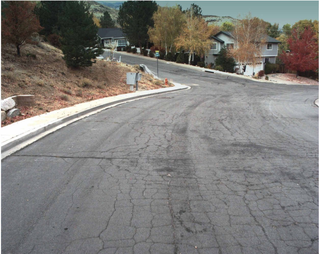
Figure 9. Pavement in Very Poor condition category (PCI 40–26).
