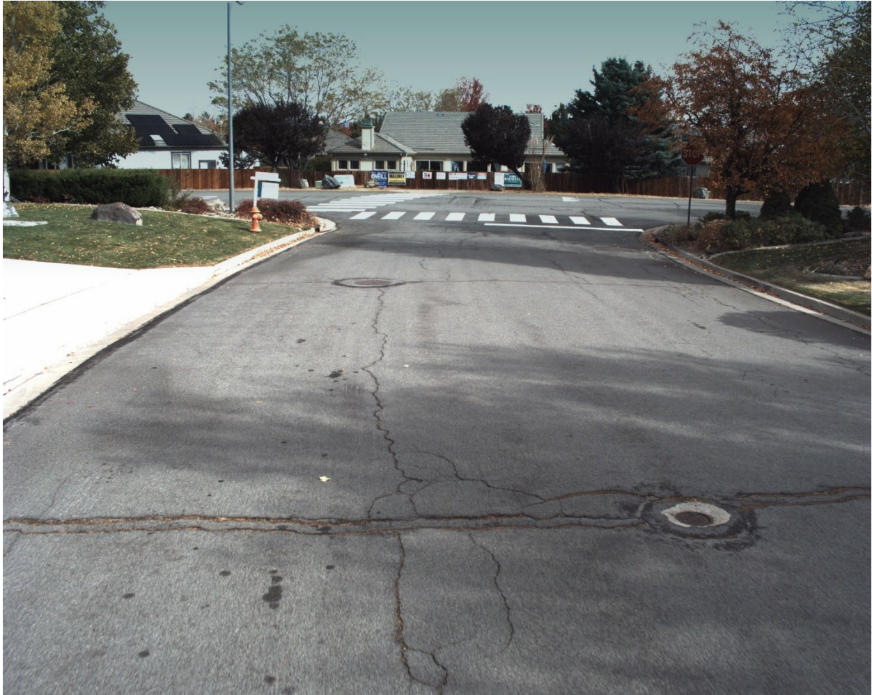
Figure 7. Pavement in Fair condition category (PCI 70–56).
