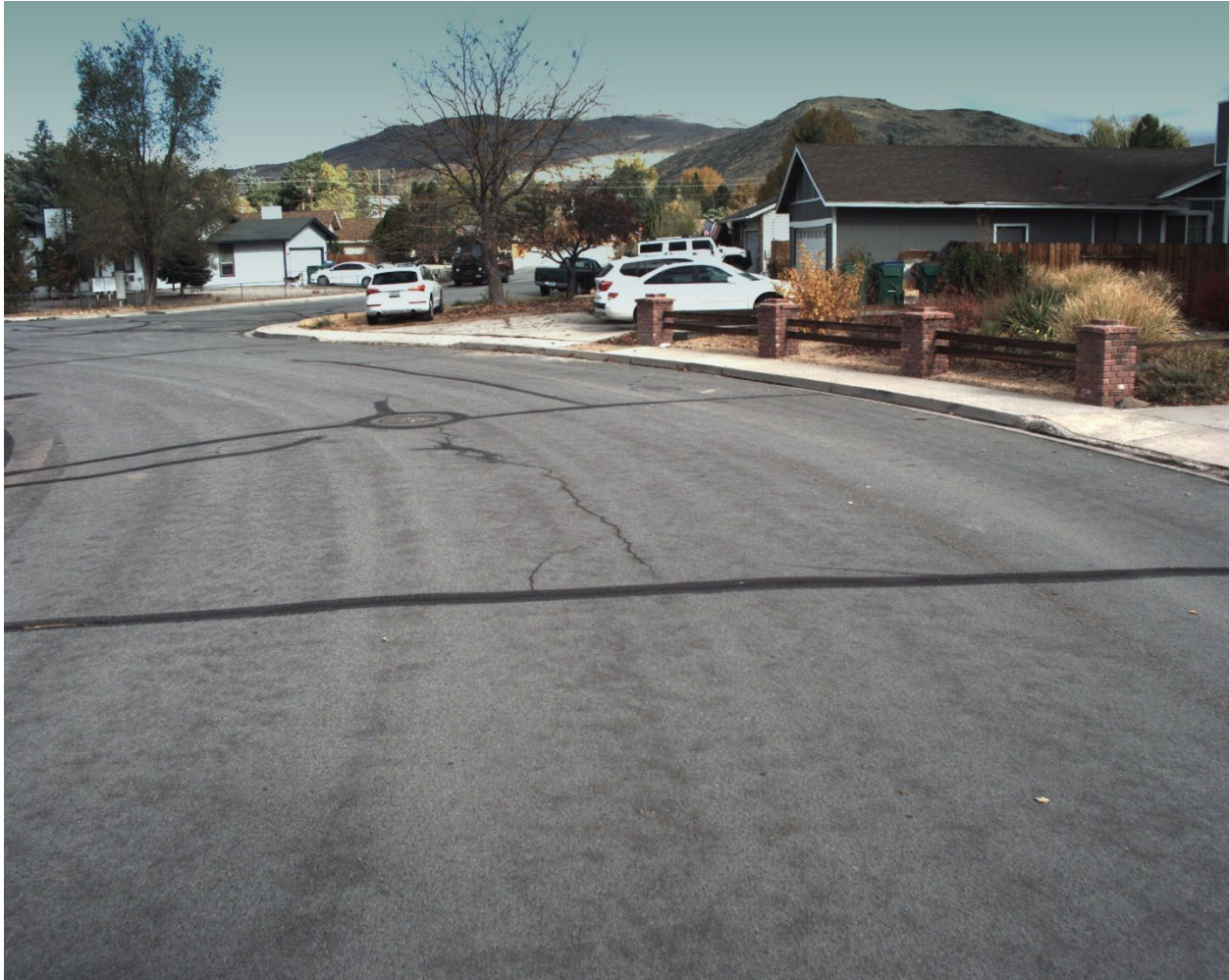
Figure 6. Pavement in Satisfactory condition category (PCI 85–71).
