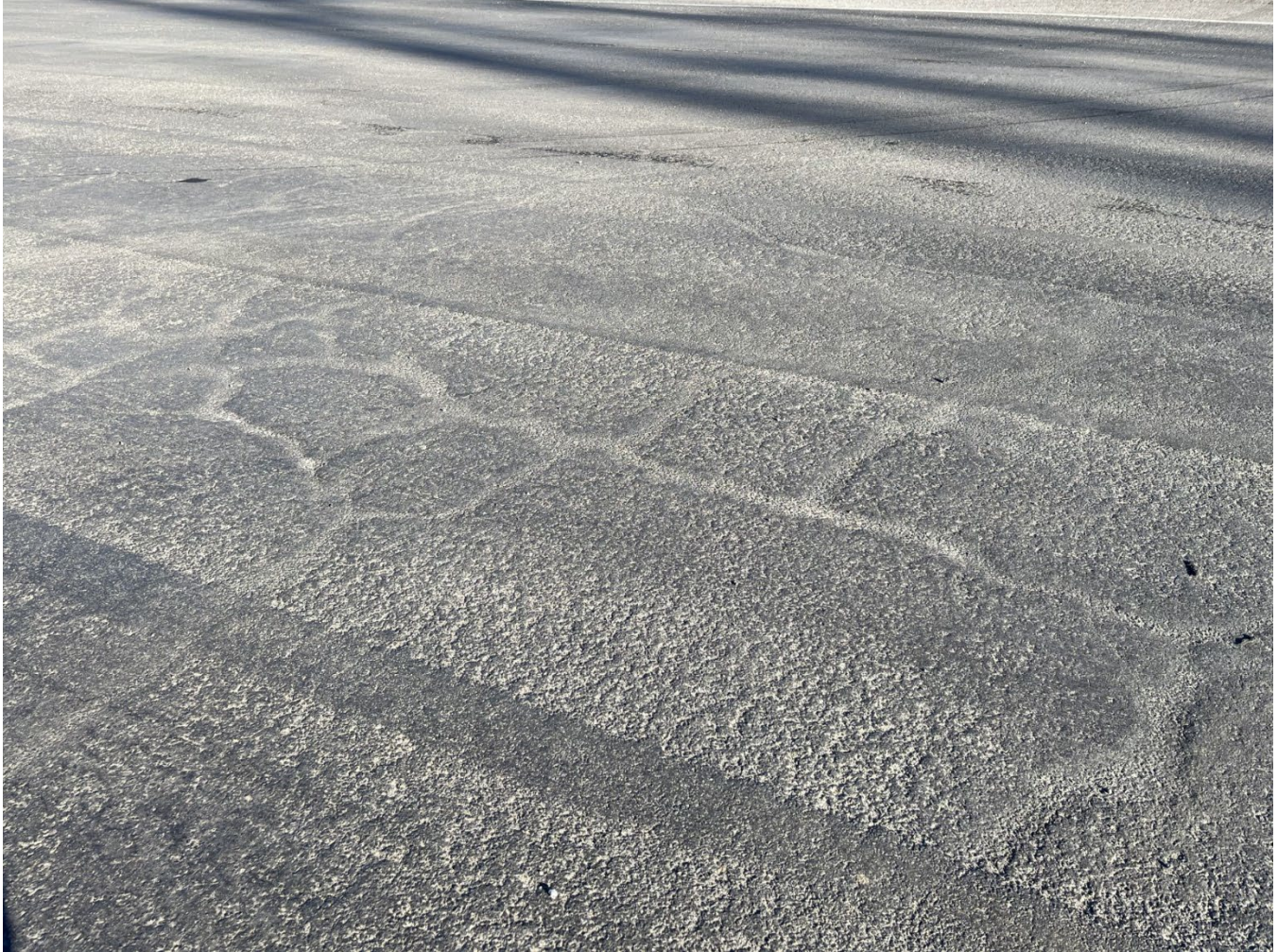
Figure 5. Mastic sealant performance in the Carson City Public Works yard (2026).
