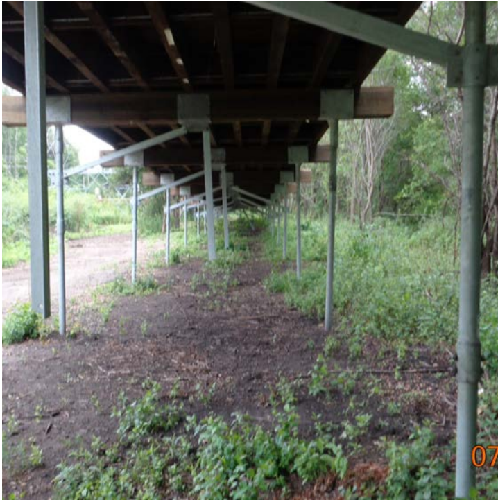
Left: The image illustrates the helical anchor structural support system that will be used for the boardwalks Right: Illustration of an extended span with steel I-beams as will be needed for the Metropolitan Council Regional Sewer Interceptor Crossing.
