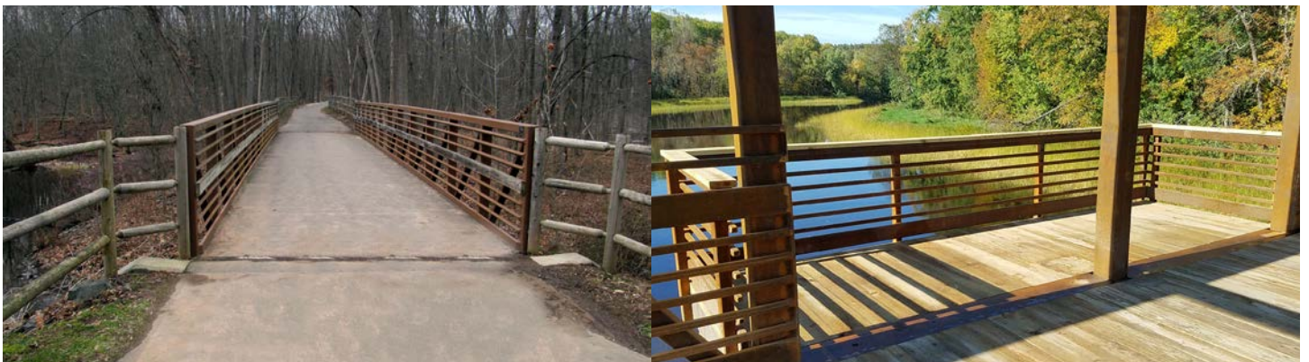
Left: The image illustrates a strategy for keeping trail users on the specified trail and out of the erodable creek bank. Right: Illustration of a look out off the side of the bridge. This could also include benches.
