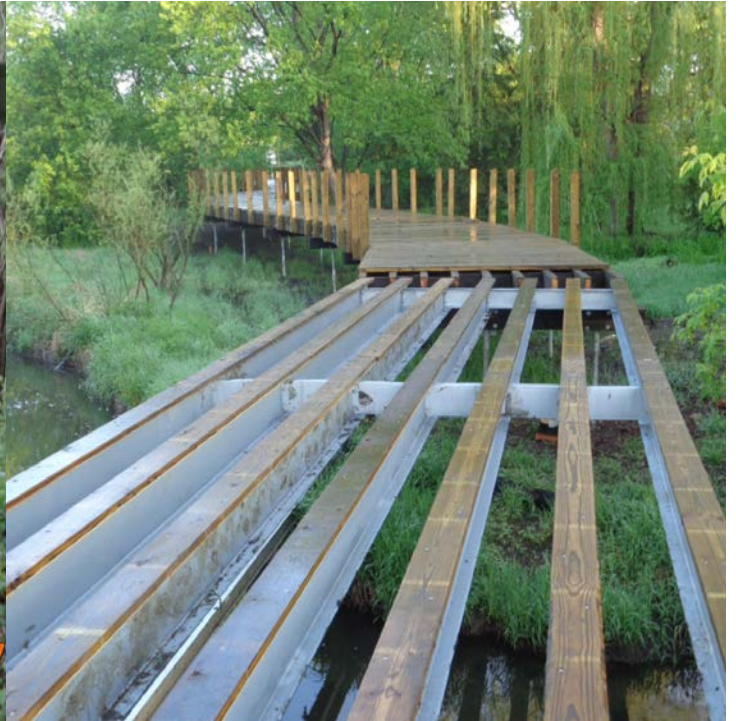
Left: The image illustrates the helical anchor structural support system that will be used for the boardwalks Right: Illustration of an extended span with steel I-beams as will be needed for the Metropolitan Council Regional Sewer Interceptor Crossing.
