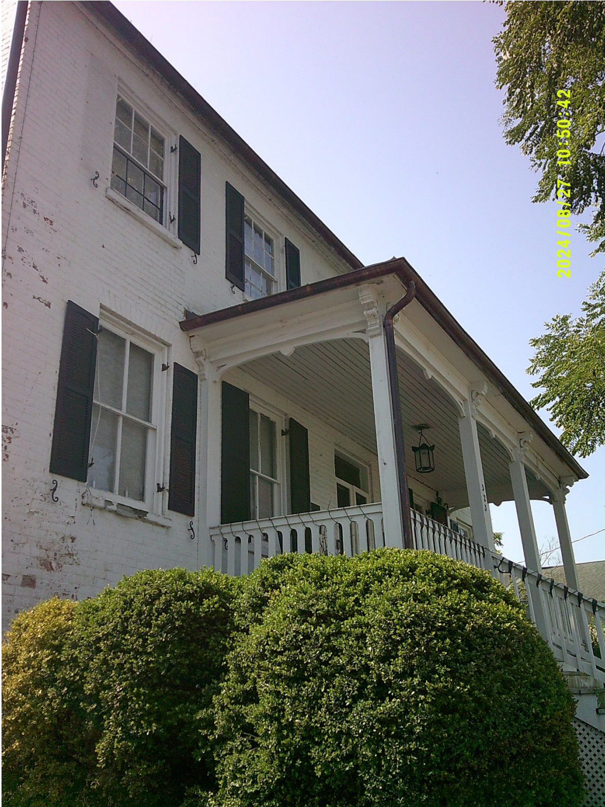
View from E. Washington Street.
