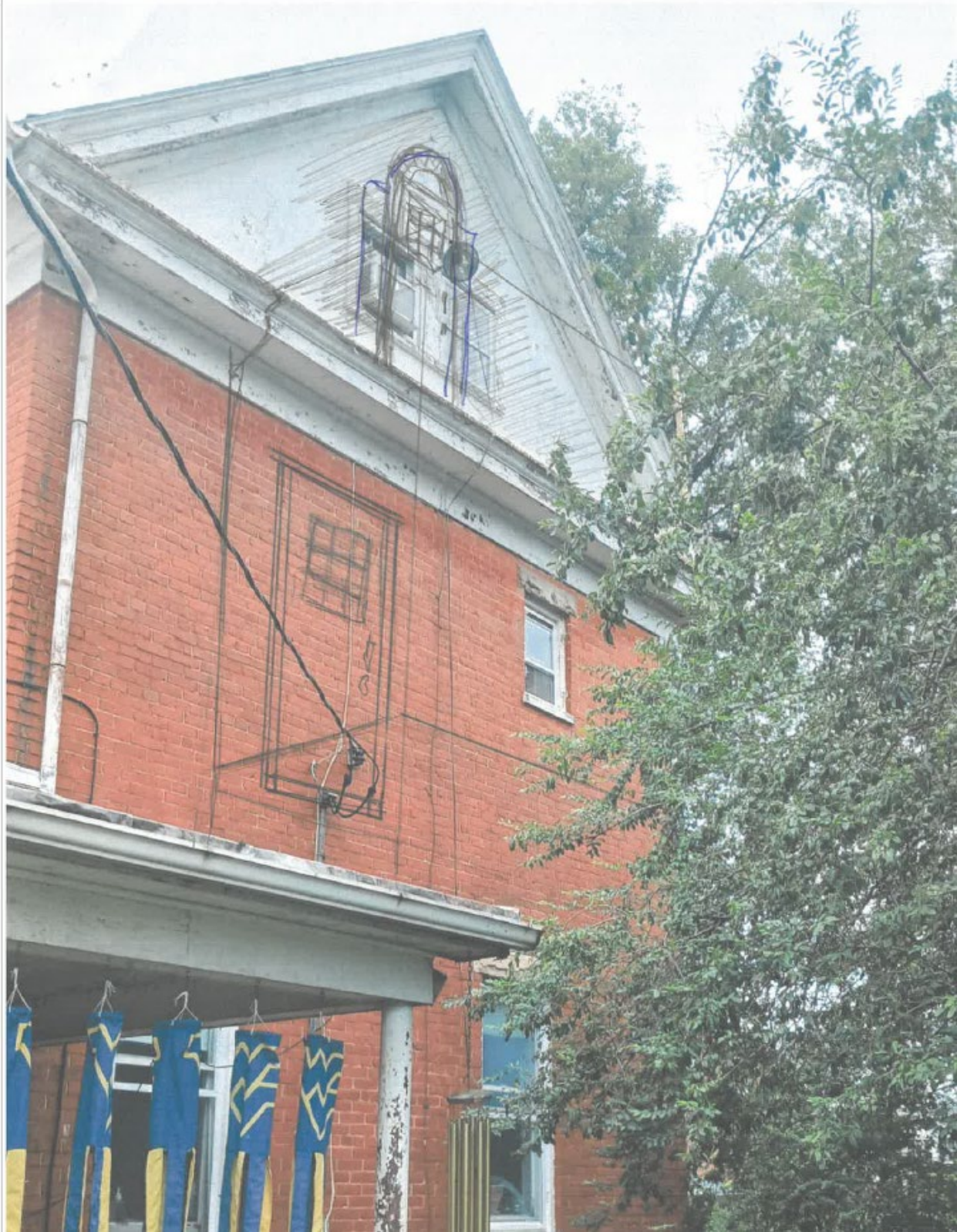
DECK – View of the rear of the property with proposed doors to 2 nd and 3 rd floor decks
