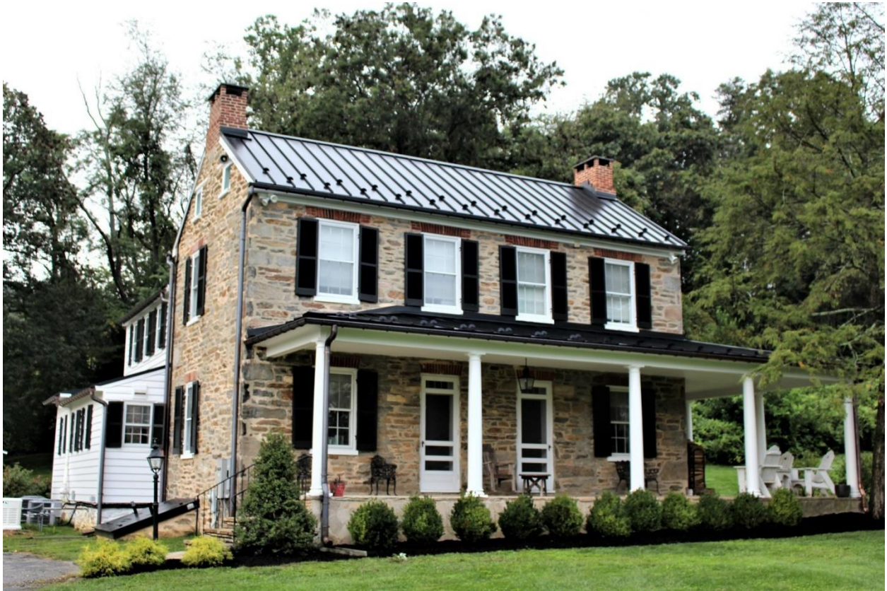
IMAGE 9 Standing Seam Metal Roof
