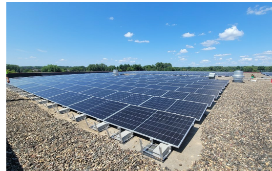
Cottage Grove Ice Arena
